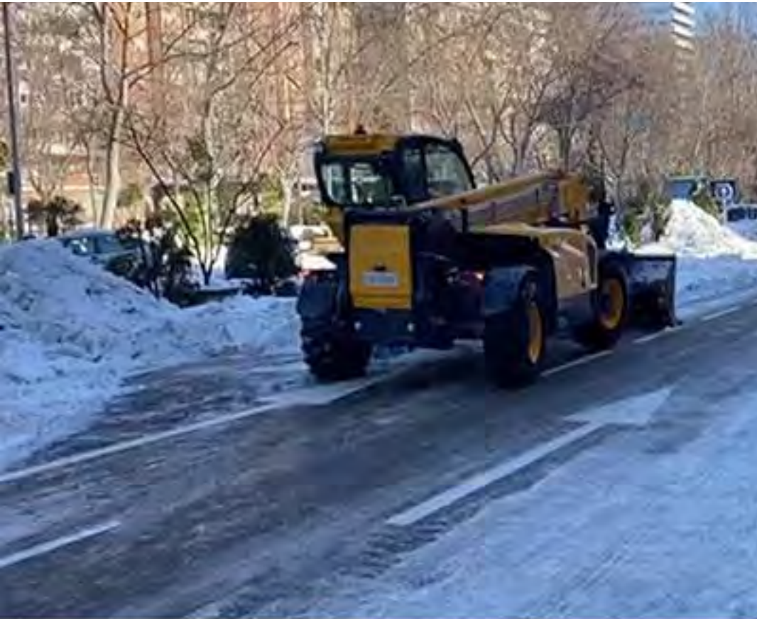
One of the streets adjacent to the Santiago Bernabeu Stadium, in Madrid, during the removal of ice and snow slabs.
