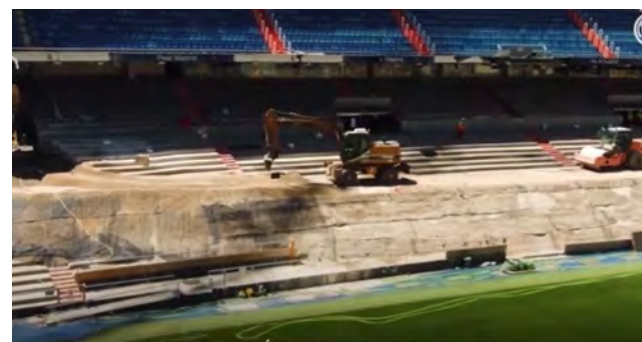
MODERNIZATION OF THE STADIUM'S FACILITIES
