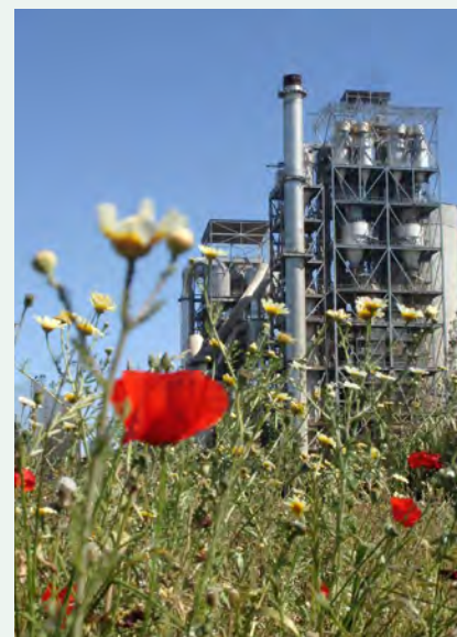
The Cementos Portland Valderrivas Group's cement factory in Alcalá de Guadaíra (Seville) began operations in 1964.
